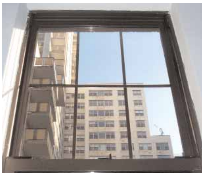
The forgotten market: existing windows
