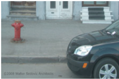
©2008 Walter Sobkow Architects Windows are not the only elements maligned by inappropriate replacements.
