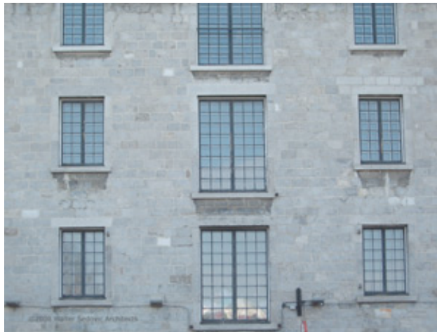
Traditional storm window systems offer not only superior performance and energy efficiency, but can also be a graceful complement to the historic sash.
